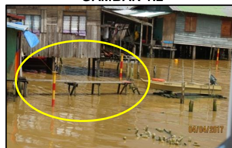
Pelabuhan Sandakan Oil Jetty - Protection Barrier at Sg. Mowtas (04.04.2017)
