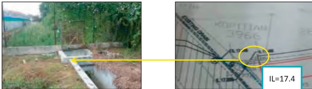
Earth Drain - Invert Level (IL) (11.01.2018)
