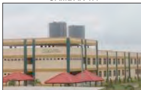
Bahagian Atas Blok Asrama SMSTG - Dua (2) Unit Elevated Water Tank (24.12.2017)
