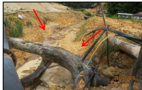
Lot 1573 Grn 74691, Lot 1574 Grn 74695, Lot 1575 Grn 74696 dan Lot 1576 Grn 74697 Mukim Pantai, Seremban - Kerosakan Tebing Sungai (28.11.2016)
