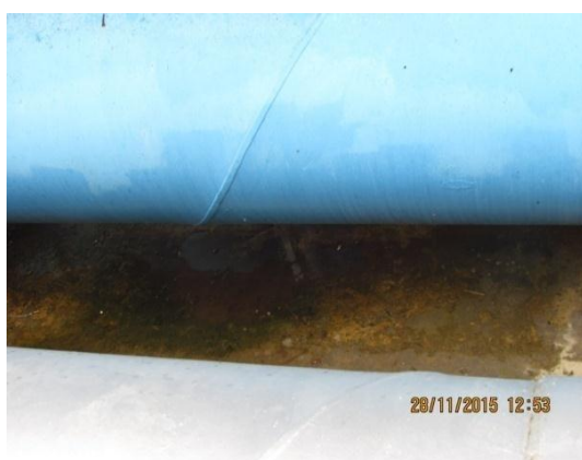
Gambar 3.5 Kebocoran di Tangki Sand Filter
