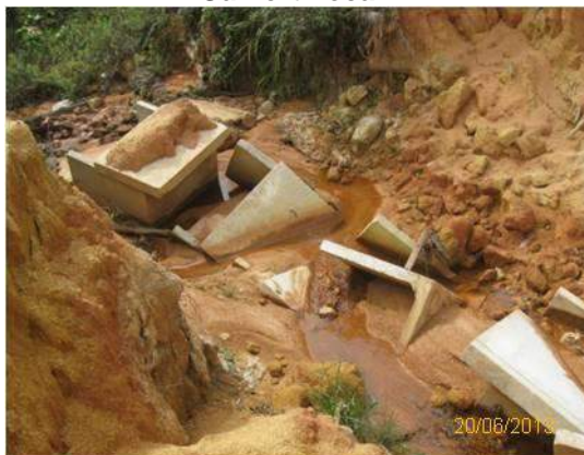
Gambar 1.5 Culvert Pecah
