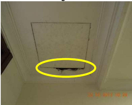
Gambar 1.9 Siling Pecah
