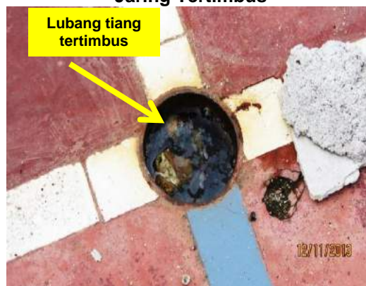
Gambar 3.2 Lubang Tiang Jaring Tertimbus
