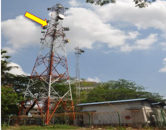
Gambar 4.3 Menara Jenis 4 Legged YTL Communication Sdn. Bhd.
