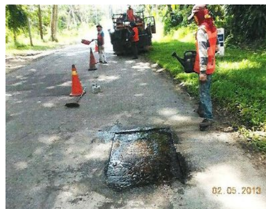
Gambar 1.15 Penampalan Pothole Dilaksana
