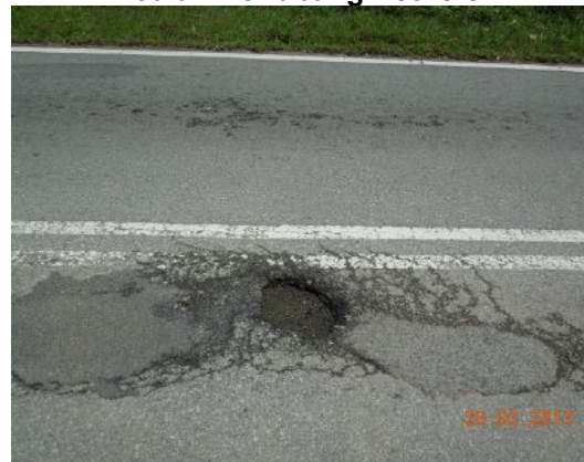
Gambar 1.4 Jalan Berlubang/Pothole
