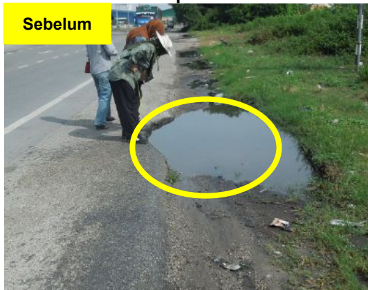
Gambar 1.21 Lubang/ Pothole Berukuran 50mm Di Tepi Jalan
