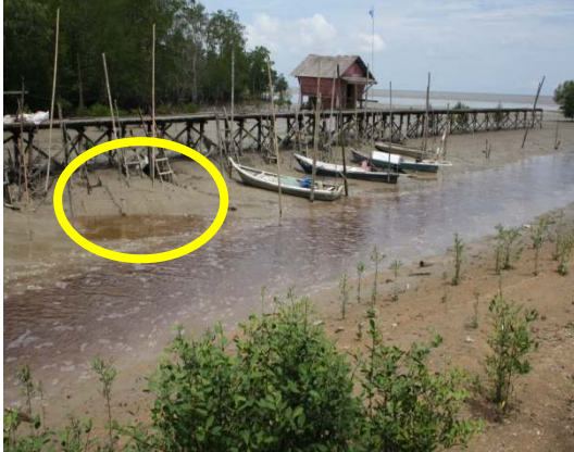
Gambar 3.3 Tebing Sungai Mengalami Proses Hakisan
