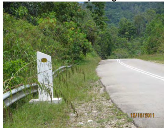
Gambar 3.32 KM Post Baru Dipasang Rosak
