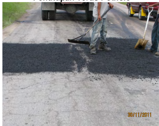
Gambar 3.18 Penutupan Terus Pothole
