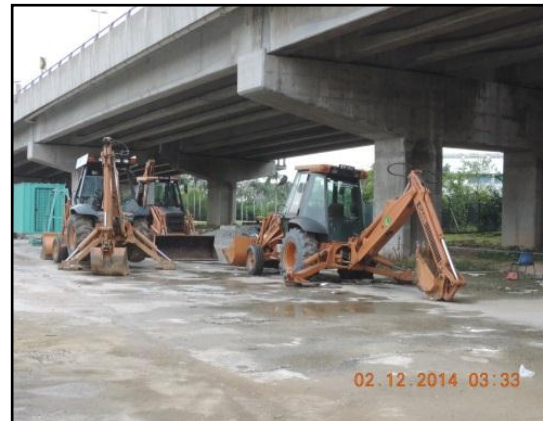
GAMBAR 13.7 Backhoe Loader menggantikan Truck Mounted Mobile Crane
