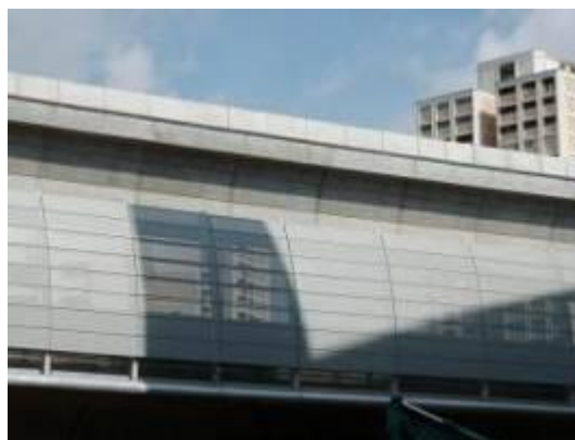
Chart 7-36 Perforated Mesh Screen Used in Singapore MRT Jurong Line
