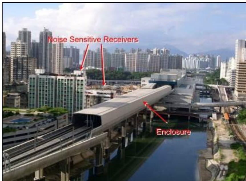
Chart 7-31 Full Enclosure for Noise Mitigation Adjacent High Rise Buildings (West Rail Hong Kong)
