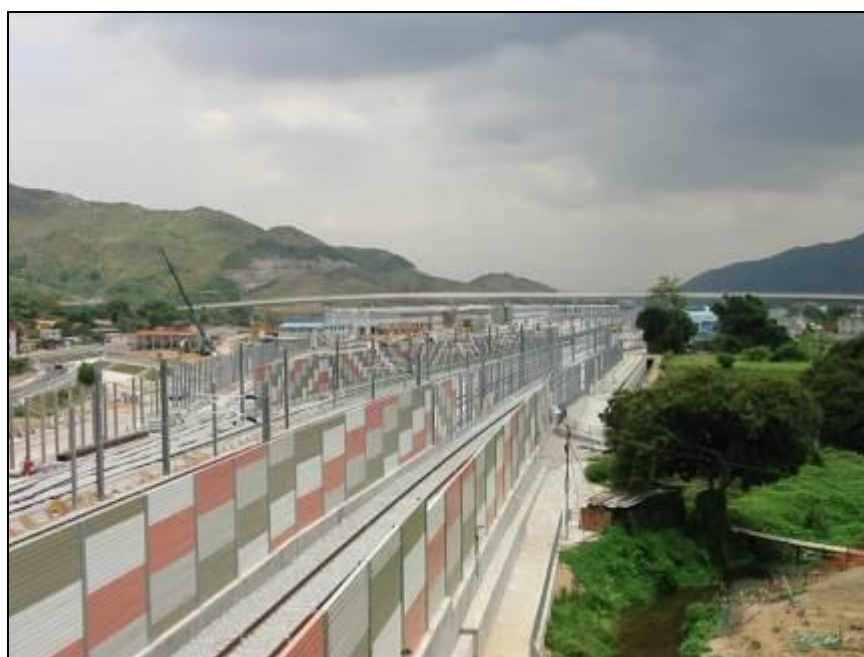
Chart 7-30 Absorptive Metal Noise Barrier (West Rail Hong Kong)
