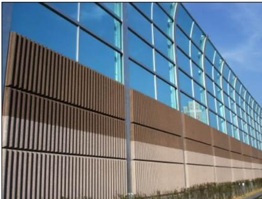
Chart 7-29 Diffusive and Reflective Transparent Noise Barrier (Diffusive panels on lower half with upper clear panels)
