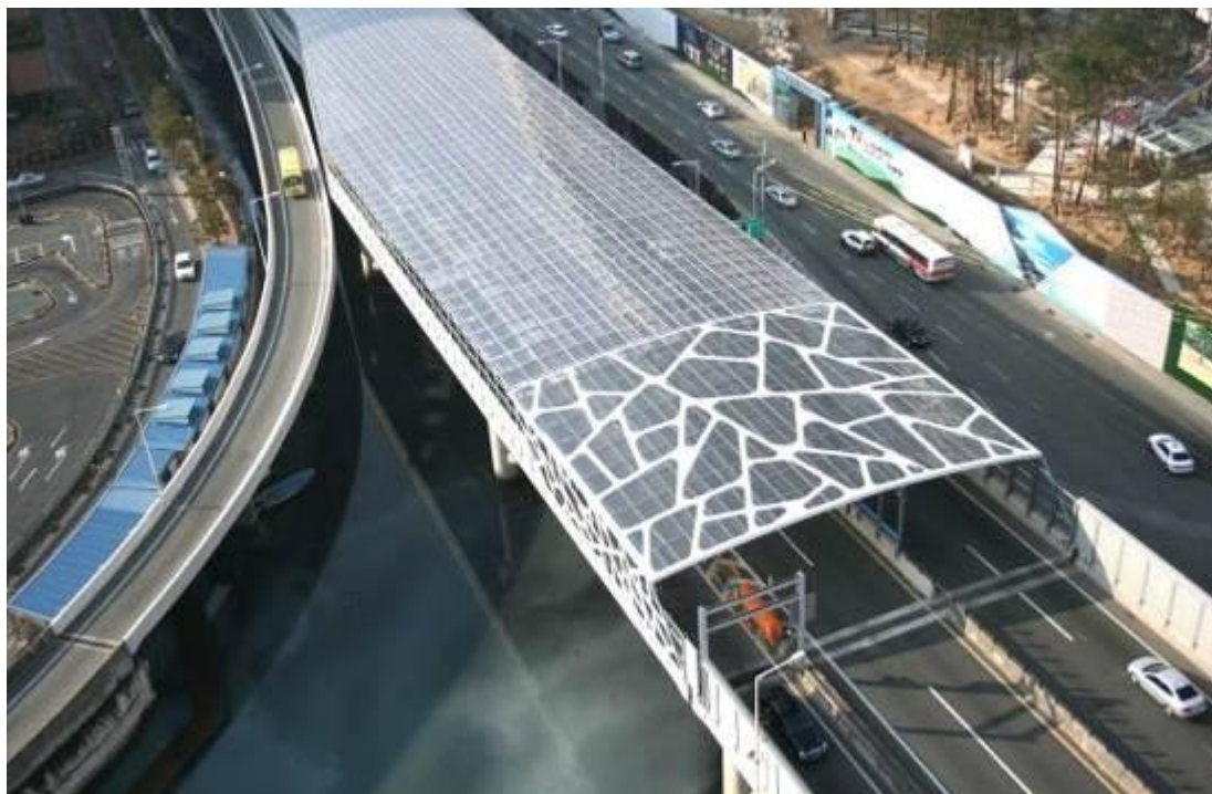
Chart 7-39 New Generation Low Visual Impact Full Enclosure
