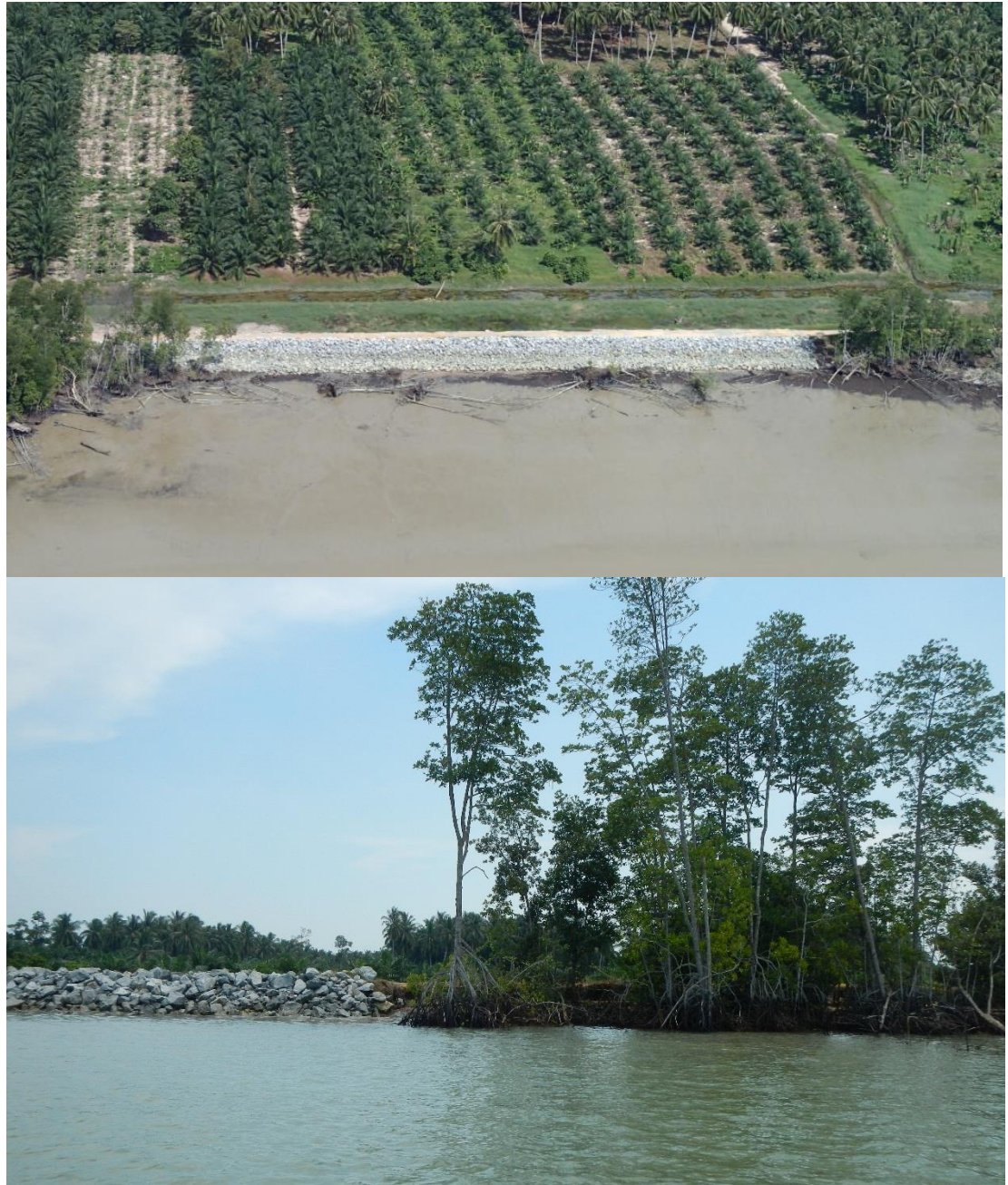
Photo 6.1 Existing coastal protection along the Piai Ramsar site – erosion of mangroves fronting the revetment are evident. Rehabilitation of these areas to restore the original hydrodynamic regime is recommended.
