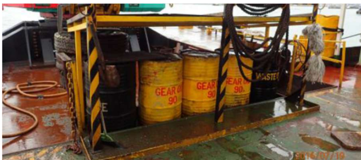
F8.18 Oil drum stored at designated covered area provided with tray
