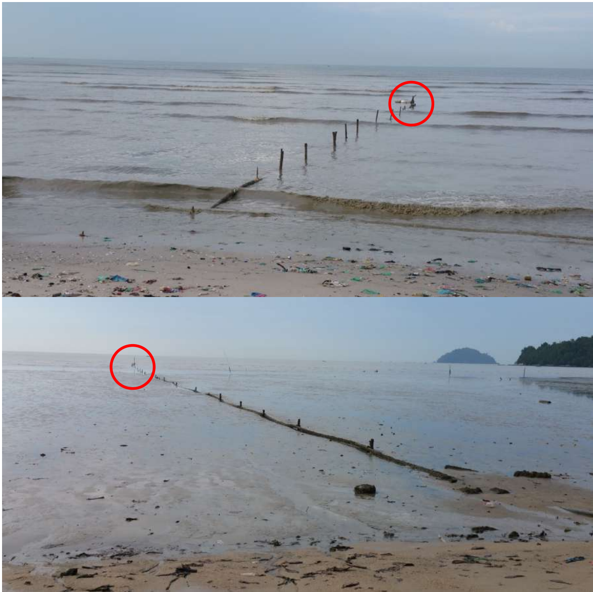
F8.29 Hatcheries seawater intake pipe found at the Project site
