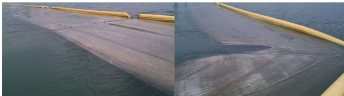
F8.8 Flaring silt curtain
