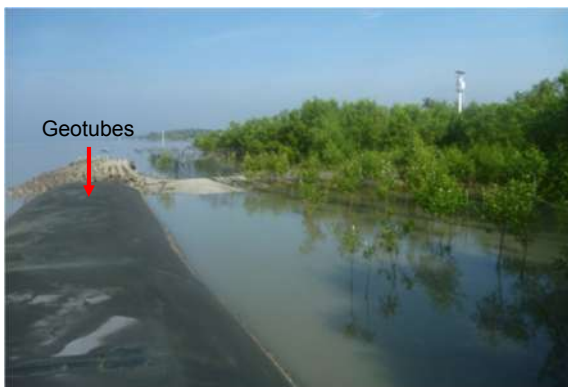
Mangrove development behind geotubes at Sungai Hj. Dorani (after 7 years)
