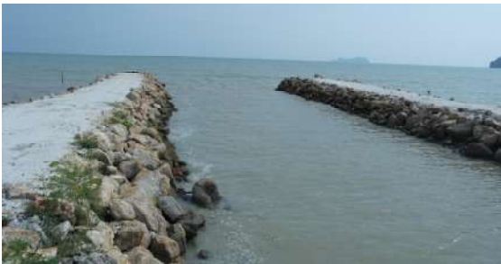
F5.14 River training structure at Bayan Lepas Main Drain outlet
