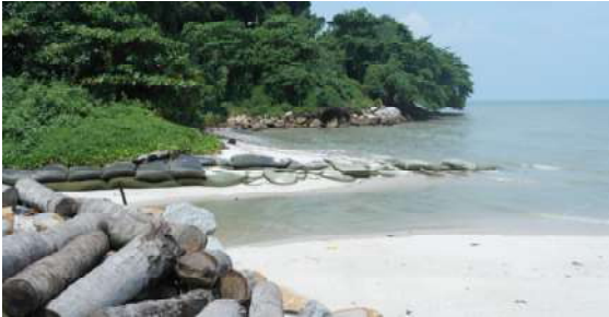
F5.22 Sand-filled geotextile bags as river training walls at Sungai Teluk Kumbar river mouth
