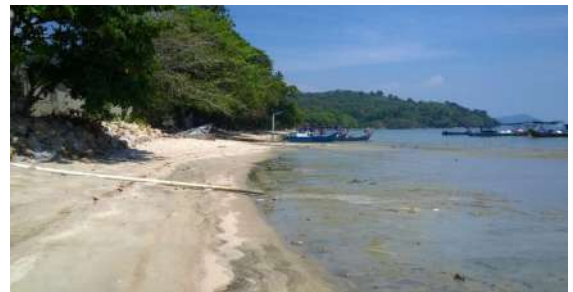
F5.27 A pipe discharging directly into the sea
