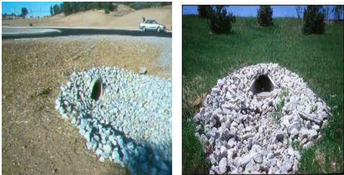
Figure 9.2 : Drainage Outlet Protection (using rock outlet protection)
