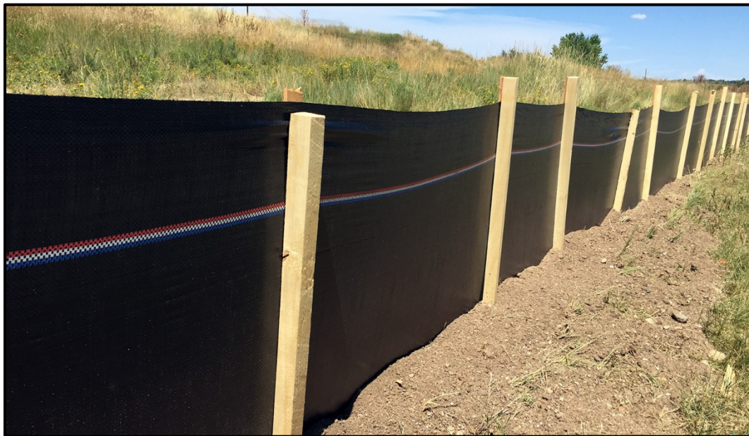
Plate 8-4: Silt Fence
