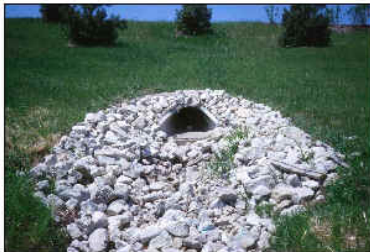
Plate 8-3: Rock Outlet Protection
