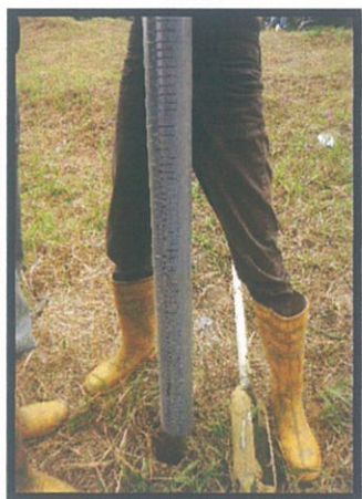
Photo 21: installation of Standpipe Piezometer at GW7
