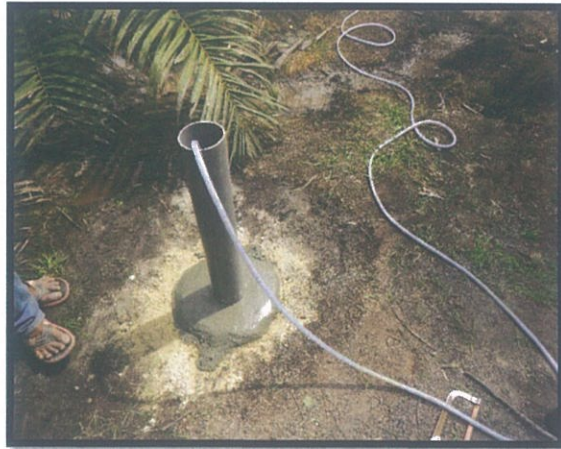
Photo 6: Installation of Standpipe Piezometer
