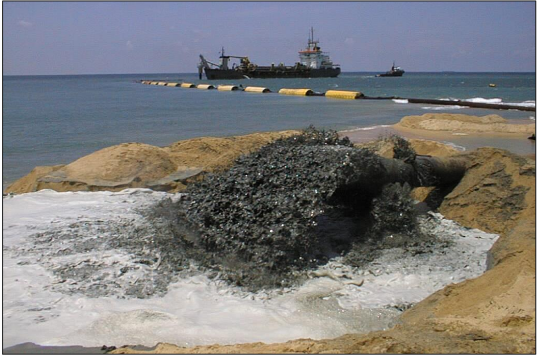
Photo 5.1 Hydraulic pumping of sand through floating pipeline.
