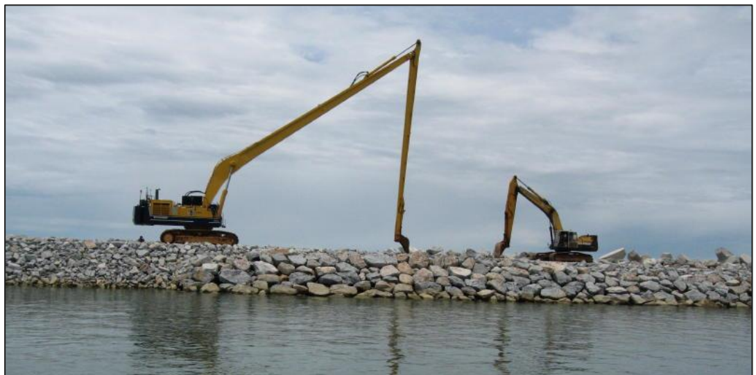
Figure 5.14 Long arm excavator for revetment construction
