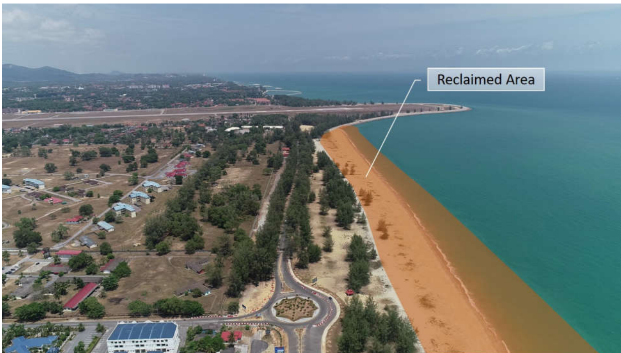
Figure 5.6: Reclaimed Area at Pantai Teluk Ketapang
