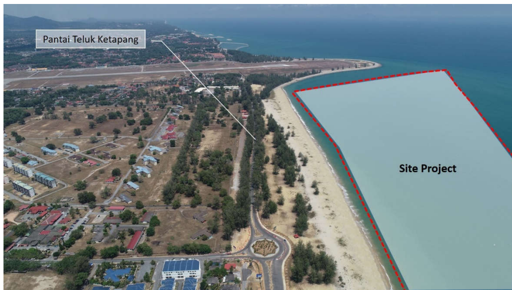
Figure 4.27: Aerial view of Pantai Teluk Ketapang
