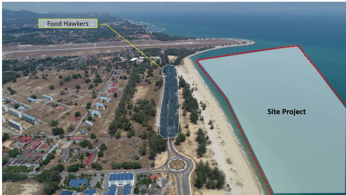
Figure 5.4: Proposed project may affect the scenic drive along Jalan Pantai Teluk Ketapang
