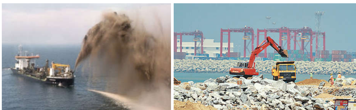
Figure 5.1: Reclamation Work in Progress
