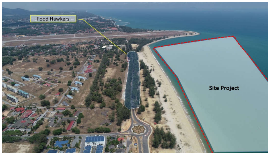
Figure 5.10: Proposed project may affect the scenic drive along Jalan Pantai Teluk Ketapang
