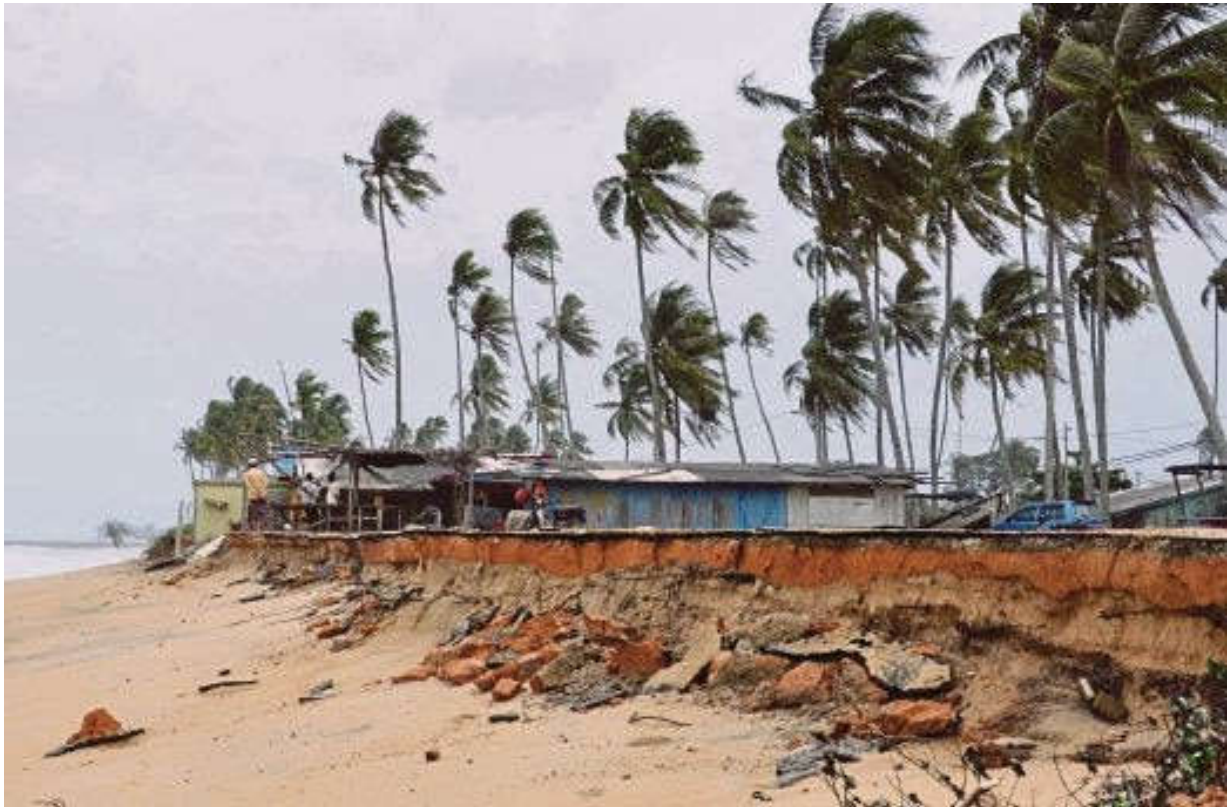
Figure 5.5: Coastal Erosion at Kampung Tanjung Gelam, Mengebang Telipot
