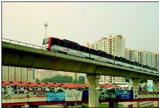
Plate 5-11 : Example of Railway Bridge (Light Rail Transit)
