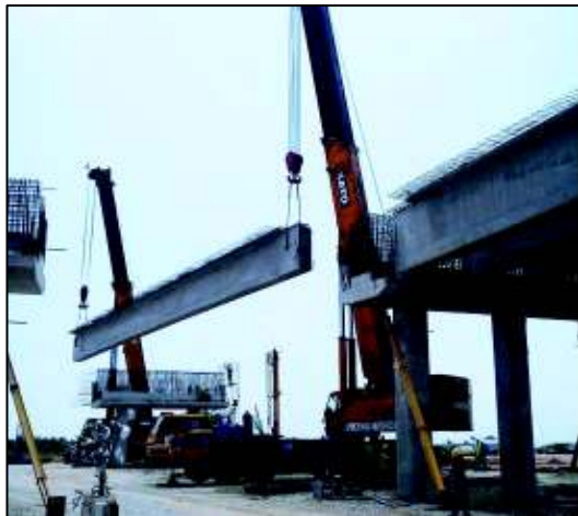
Plate 5-12 : Example of Beam Launching Using Mobile Crane
