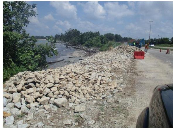
**Plate 6.2.6: Repair work was on-going along the eroded shoreline.**
