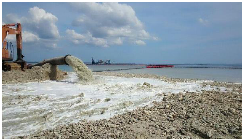
Plate 5.3.3: Discharge point of hydraulic pumped sand
