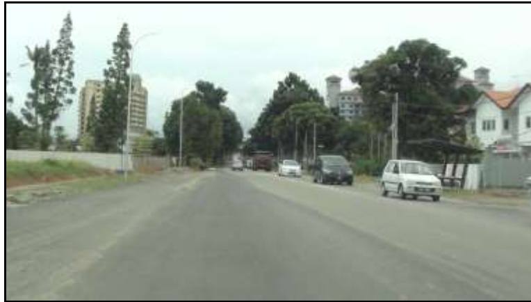
Plate 1. A view of Road FR5
