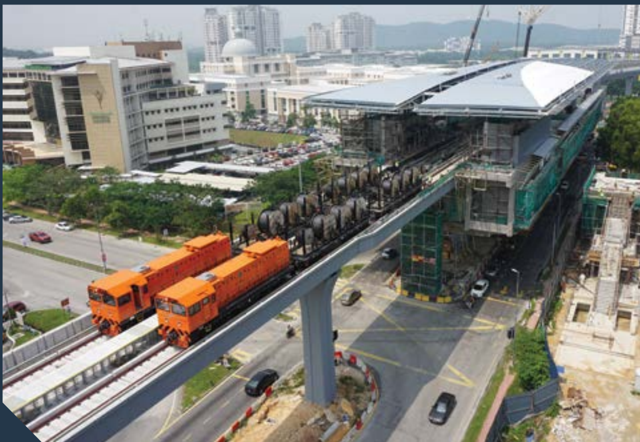
▲ GOOD VIEW: An aerial view of the Kota Damansara Station with cable installation works in progress.
