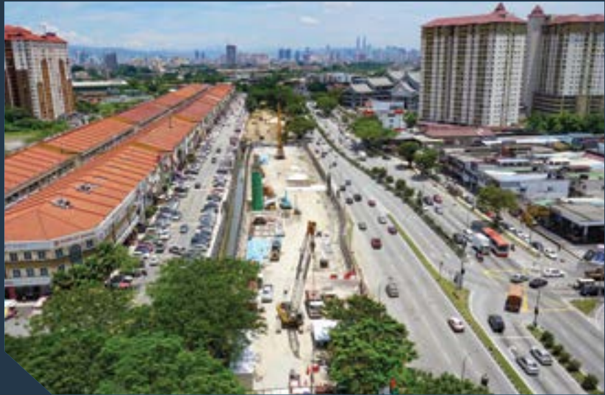
▲ INITIAL STAGE: Preparation works for test pile works at the future Kepong Baru Station site.
