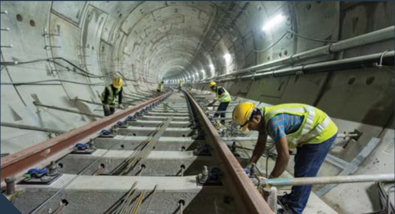
▲ HARD WORK: Workers carrying out track works inside the SBK Line tunnel.
