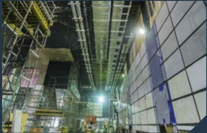
▲ IN PROGRESS: Ongoing internal cladding of the walls inside the Tun Razak Exchange Station.
