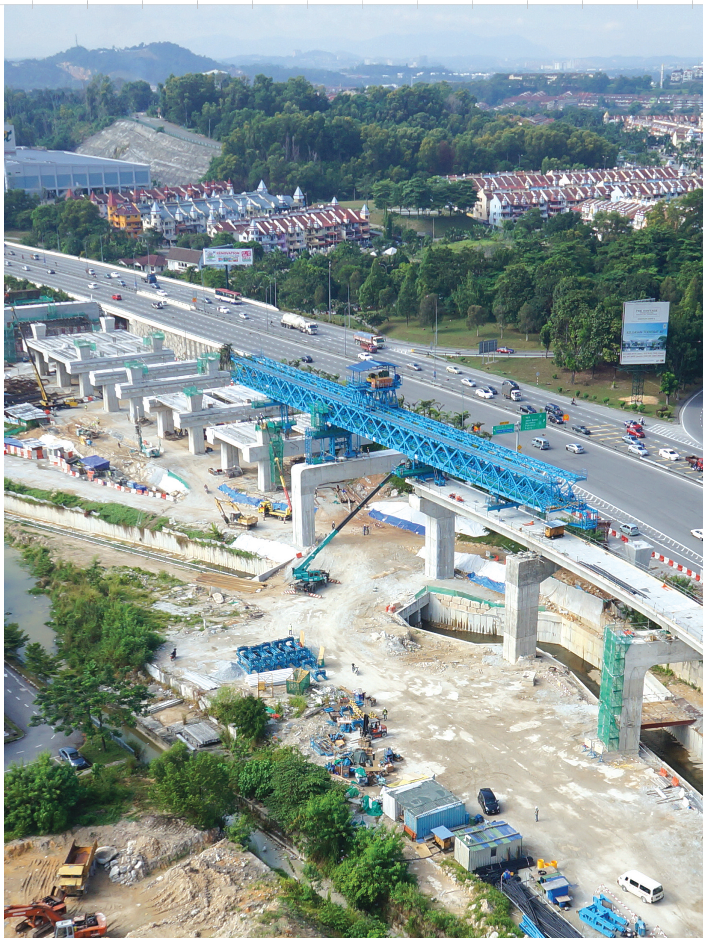
FUTURE STATION << Construction of the MRT guideway at the future Taman Sutex Station in progress.
