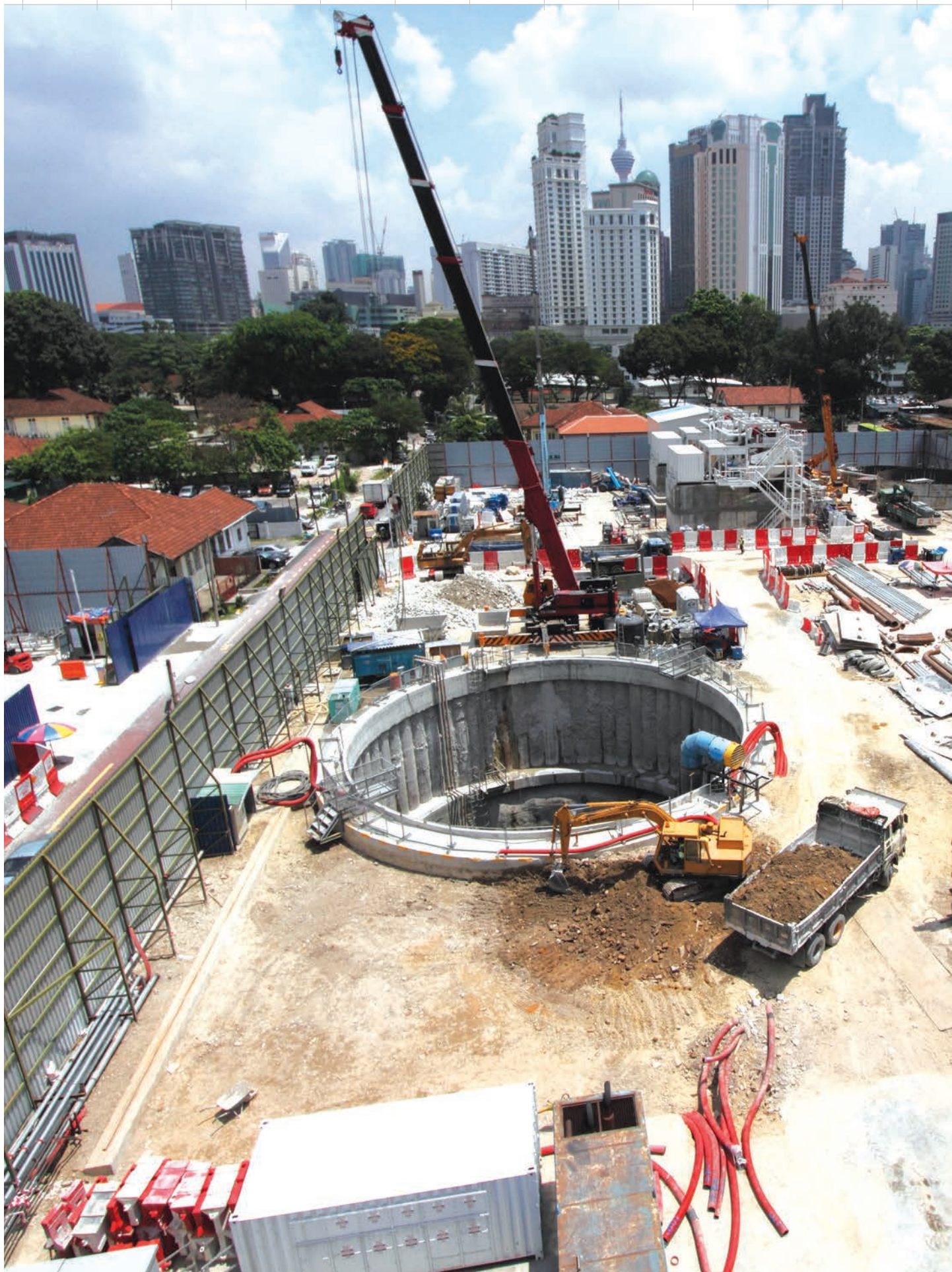
>> IN PROGRESS Aerial view of the Inai Launch Shaft.
