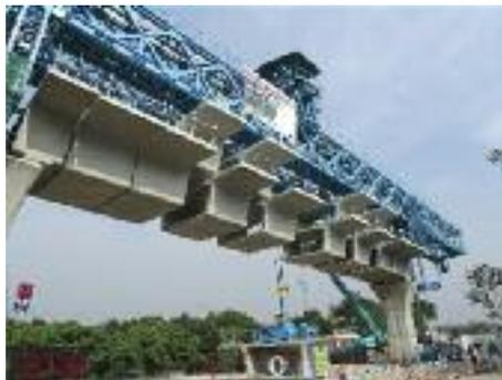
Load testing being carried out on the first launch gantry under Package V6 near Bandar Tun Hussein Onn on 9 April 2013.
