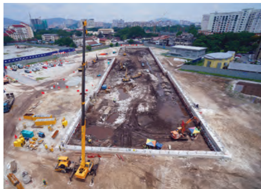
EXCAVATION The Cochrane tunnel boring machine launch shaft being prepared.
